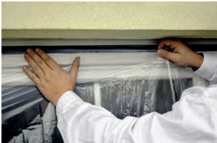
Apply dust sheet directly over tape
