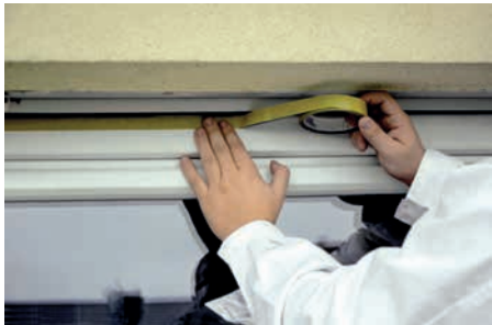
Apply tape on the surface
